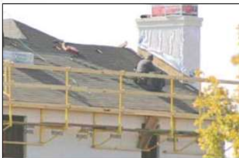
Guardrail (during construction)
